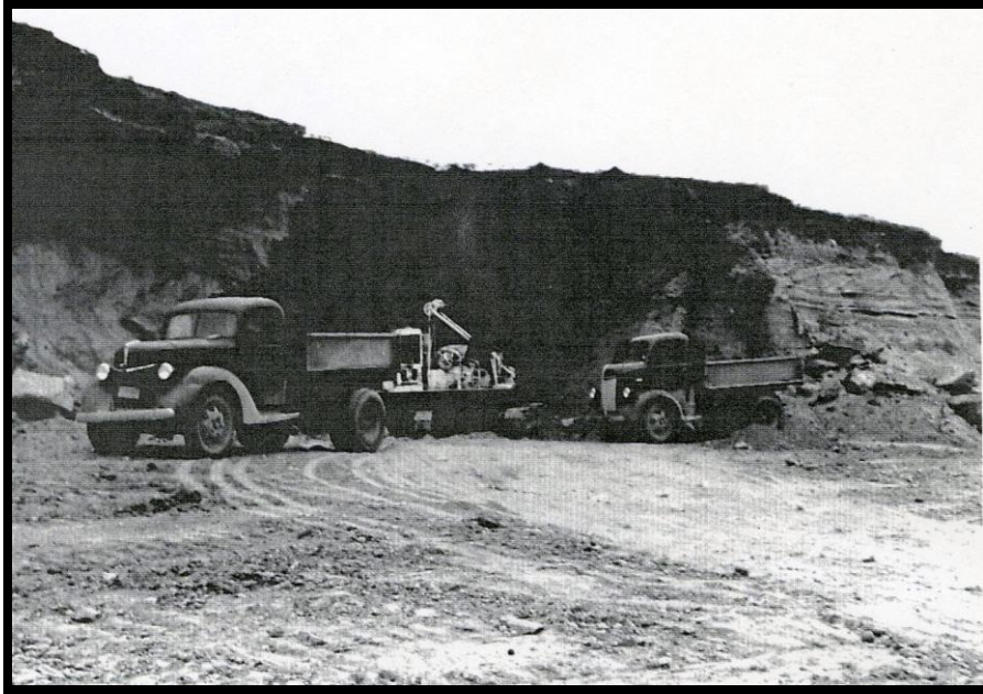
1939 Hauling Gravel from hill – Schiebe Bros Excavating
