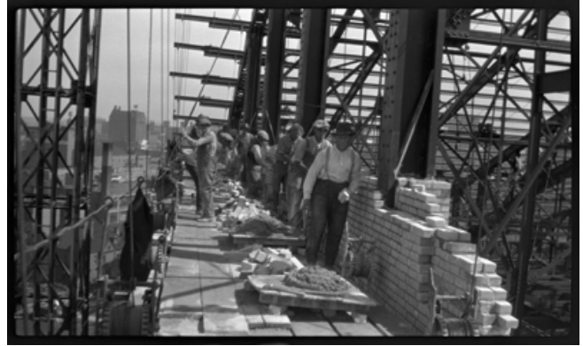
Construction Workers on Foshay
